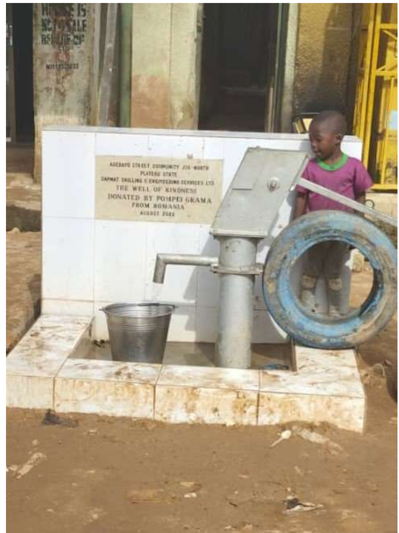
An example borehole. This one has a manual hand pump. It is our hope we have sufficient funds to install an electric pump and a 5000 liter tank at each site.
